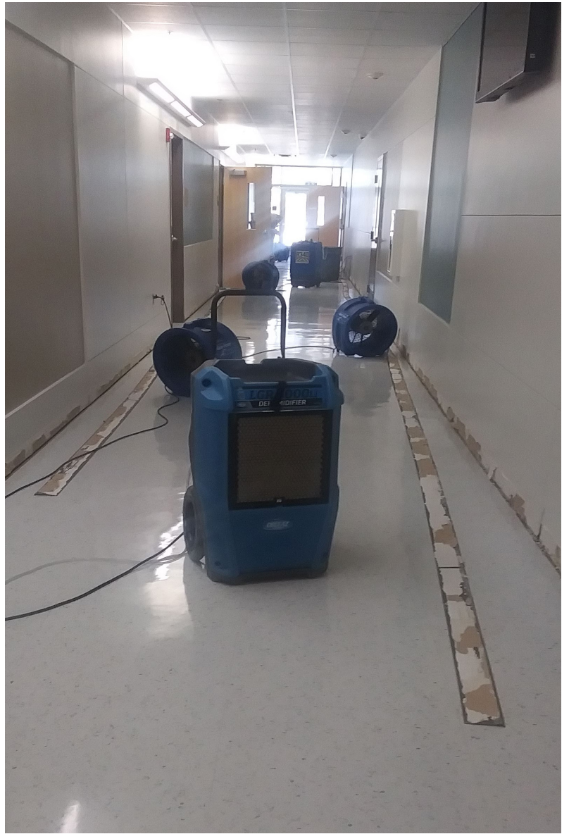
Below: Fans placed in the Arts and Communications building to dry water left by leaking pipe.
